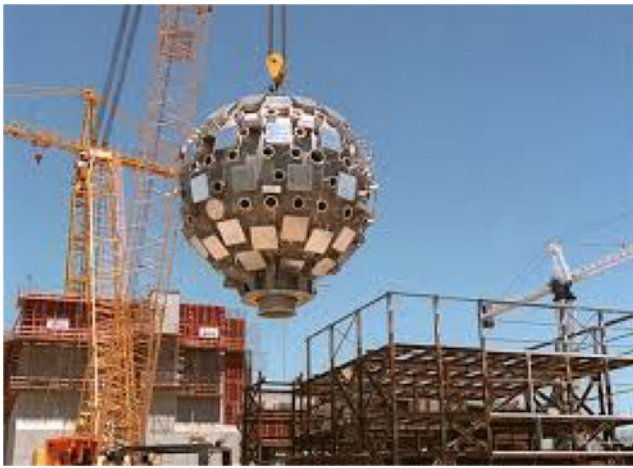
Fig. 1. Sphere of 10 m diameter at the NIF laser at the Lawrence Livermore National Laboratory LLNL in California where Laser beams are irradiated into the holes to and focused to diameters of about 100 micrometer diameter into holes of a capsule for indirect drive DT fusion in a sphere with a diameter above one millimeter producing the highest nuclear fusion gains (Hurricane et al. , 2014; Hinkel et al. , 2016).
